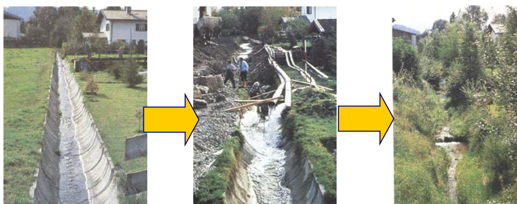
Figure 8 : Construction process for water passage naturalized.
